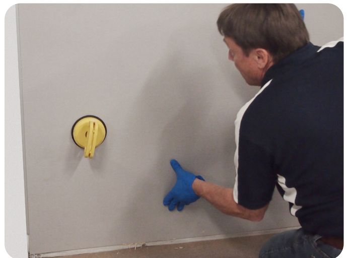
Use suction cup to fix panel.
